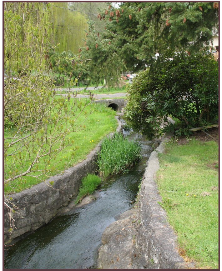
Existing Miller Creek Drainage Features - There is an opportunity to rehabilitate the creek corridor to a more natural condition.
